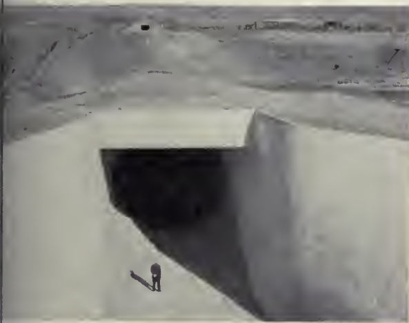
SUBWAY SYSTEM on the West Conol where water travels underground through dry Coulee siphons No. 1 and No. 2, as part of the 60-mile-long route taken by Columbo River on its way to irrigate project lands. Photo by H. E. Foss, Region 1 photographer.
